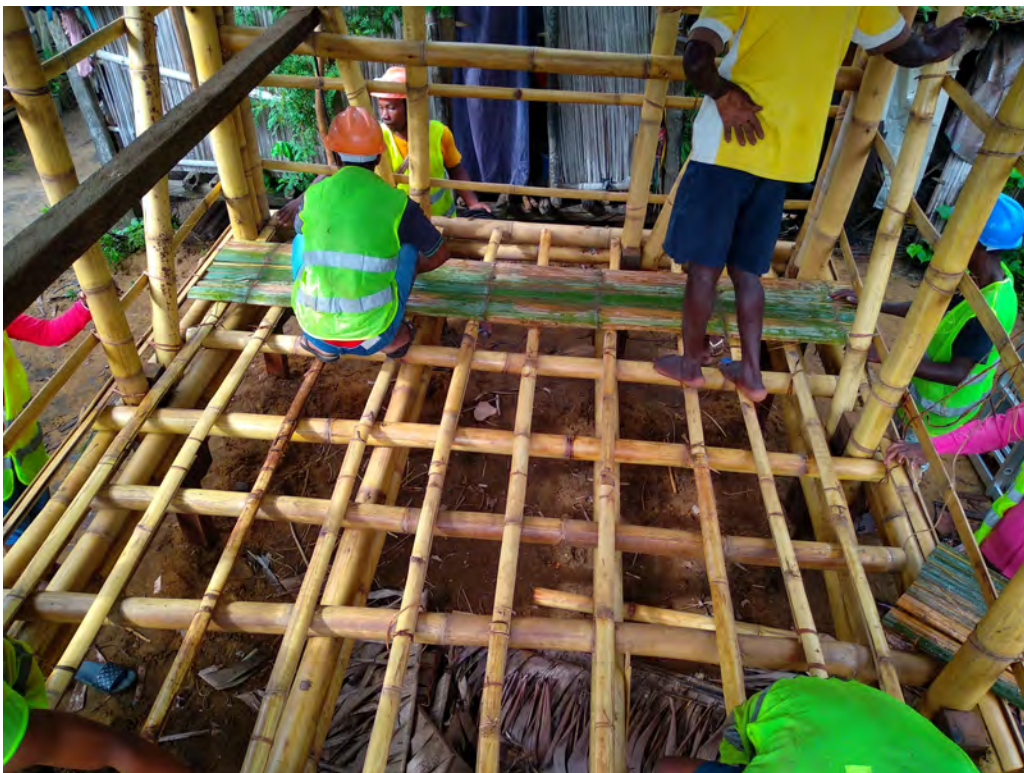
Flooring (flatten bamboo, double layer) installation
