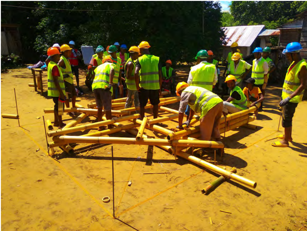
Assembly of one of the main frames
