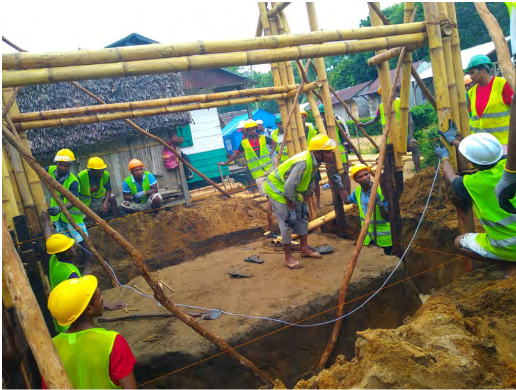
Level check when both main frames are lifted up
