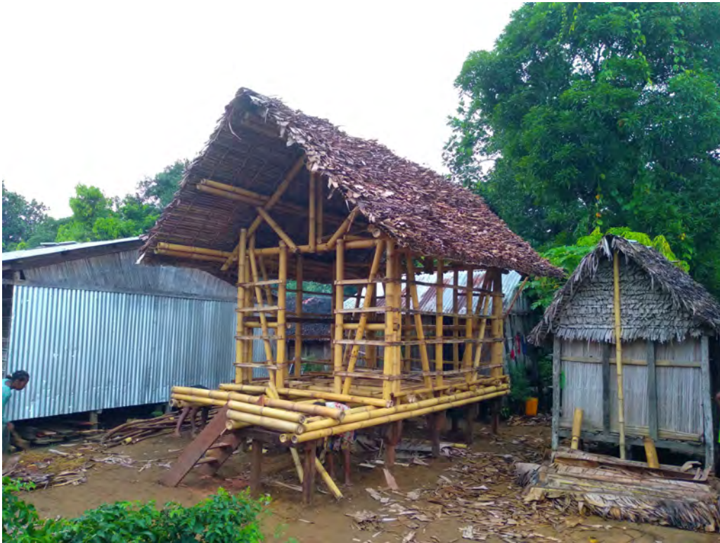
Roofing and stairs completed
