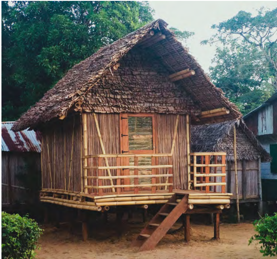
Bamboo house - Model 'B', exterior view
