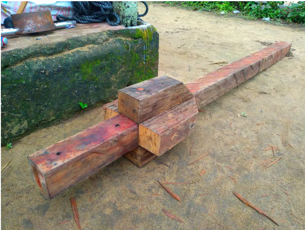
A foundation post
