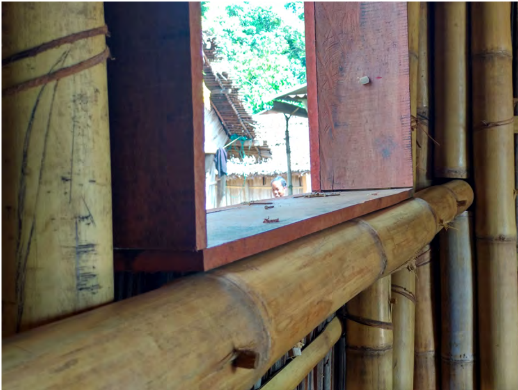
Close up of the window frame
