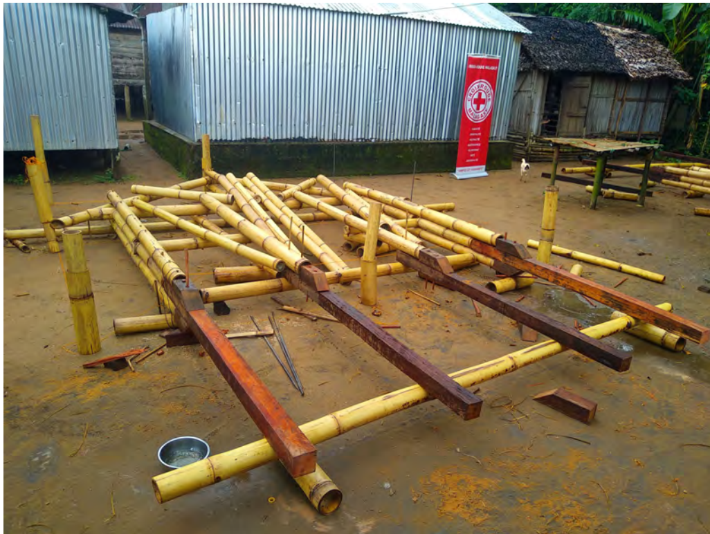
Prefabricated frame connected to foundation posts
