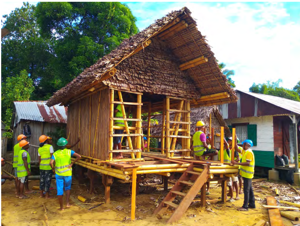
Walls, flooring and veranda in progress
