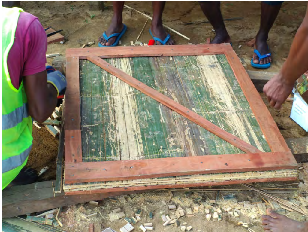
Window making in progress
