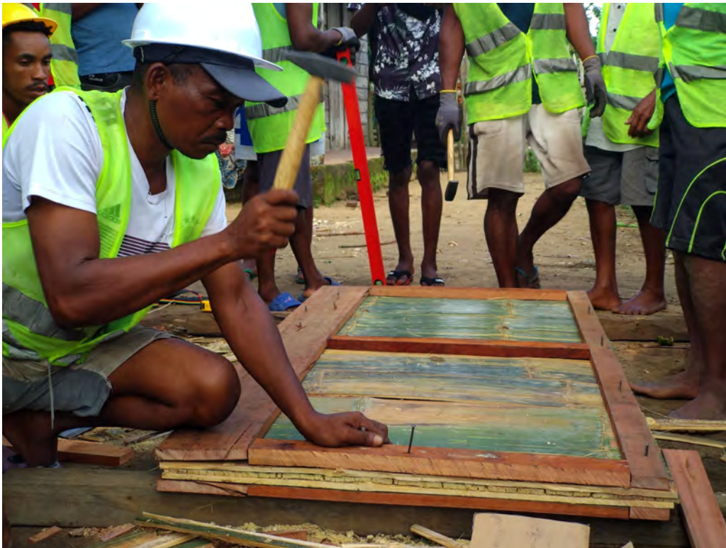
Door making in progress
