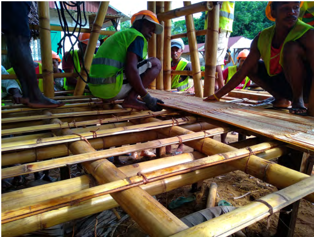
Close up of the bamboo floor slab
