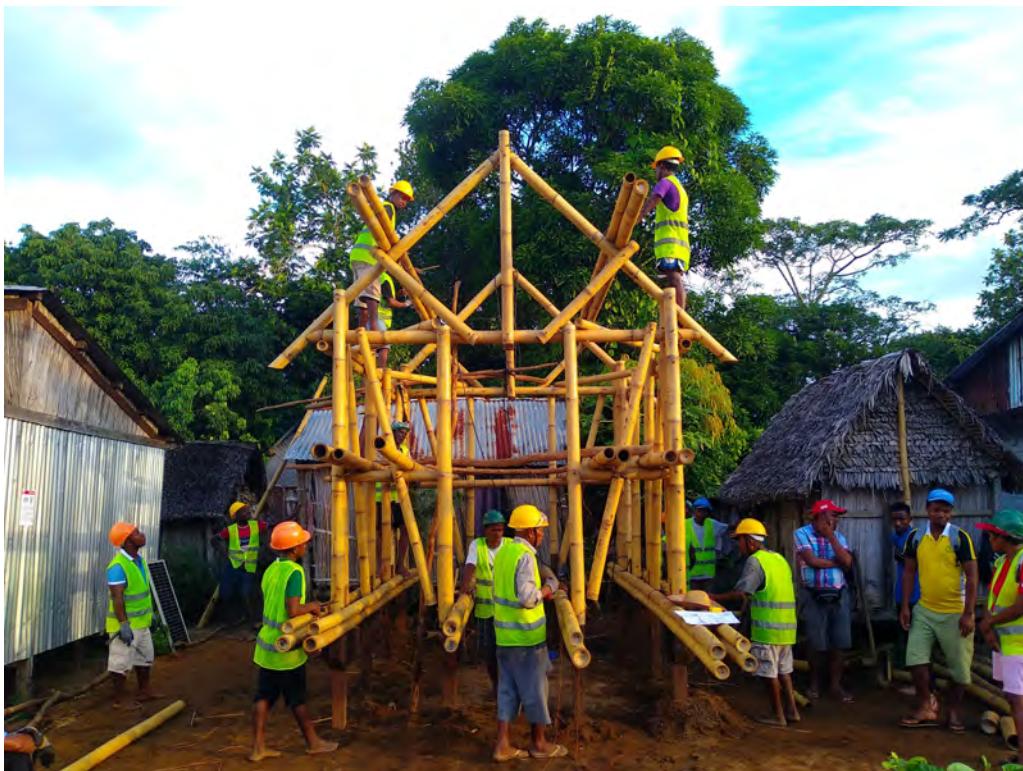
Floor beams and roof beams installation
