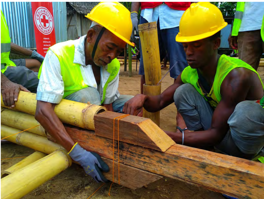
Working on the connection between columns and foundation posts
