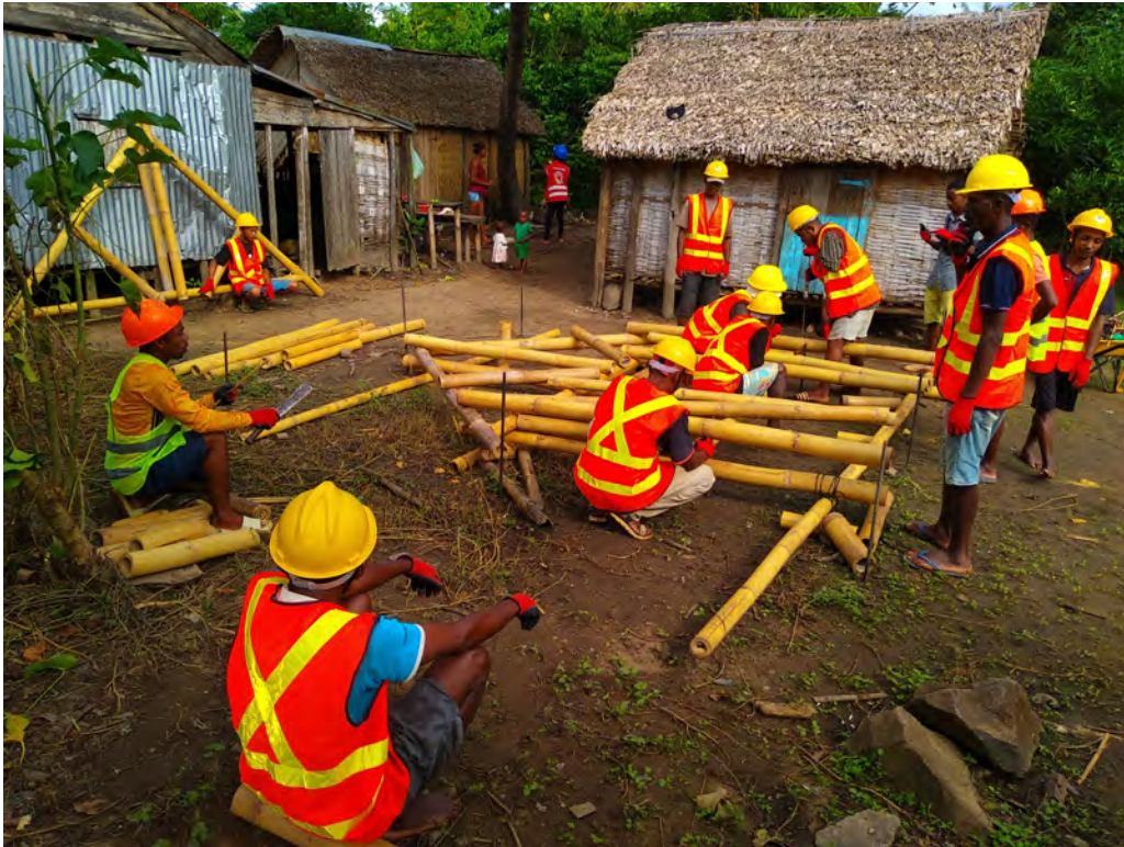
Assembling one of the prefabricated frames
