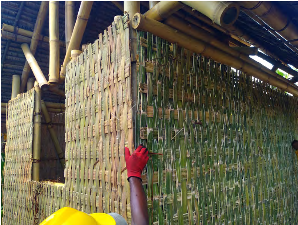
Installing the woven bamboo wall panels
