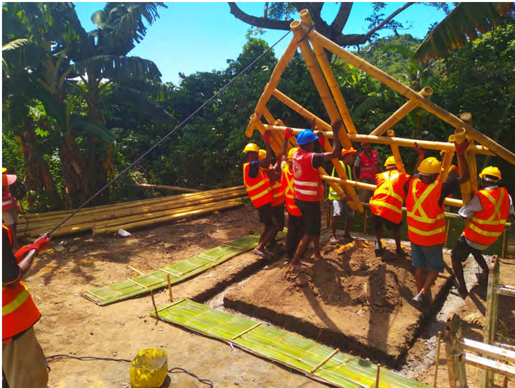
Lifting up one of the main frames
