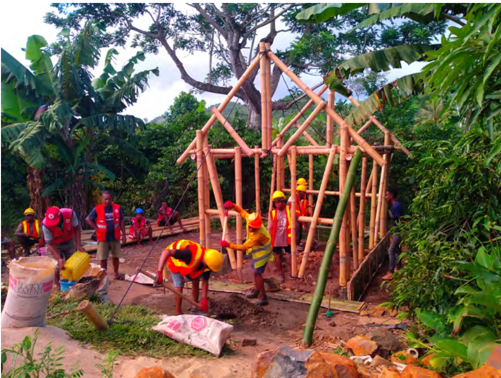
Pouring concrete for the foundation ring beam
